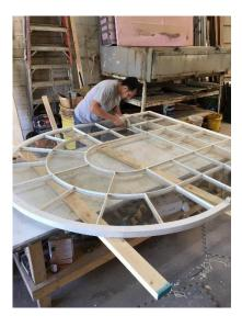
Glass is back in the transom window. Next is four coats of paint. Then it will be installed and the film applied.
